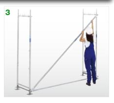
Assemble the diagonal brace with the swivel pin.
