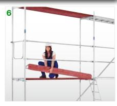
Then assemble the vertical assembly frames and the decks of the next level, click in the diagonal braces, the guardrails and the decks.
